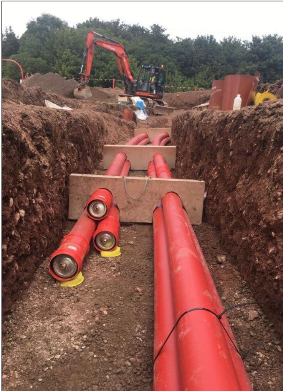
Figure 3.6: Typical Trench Construction
