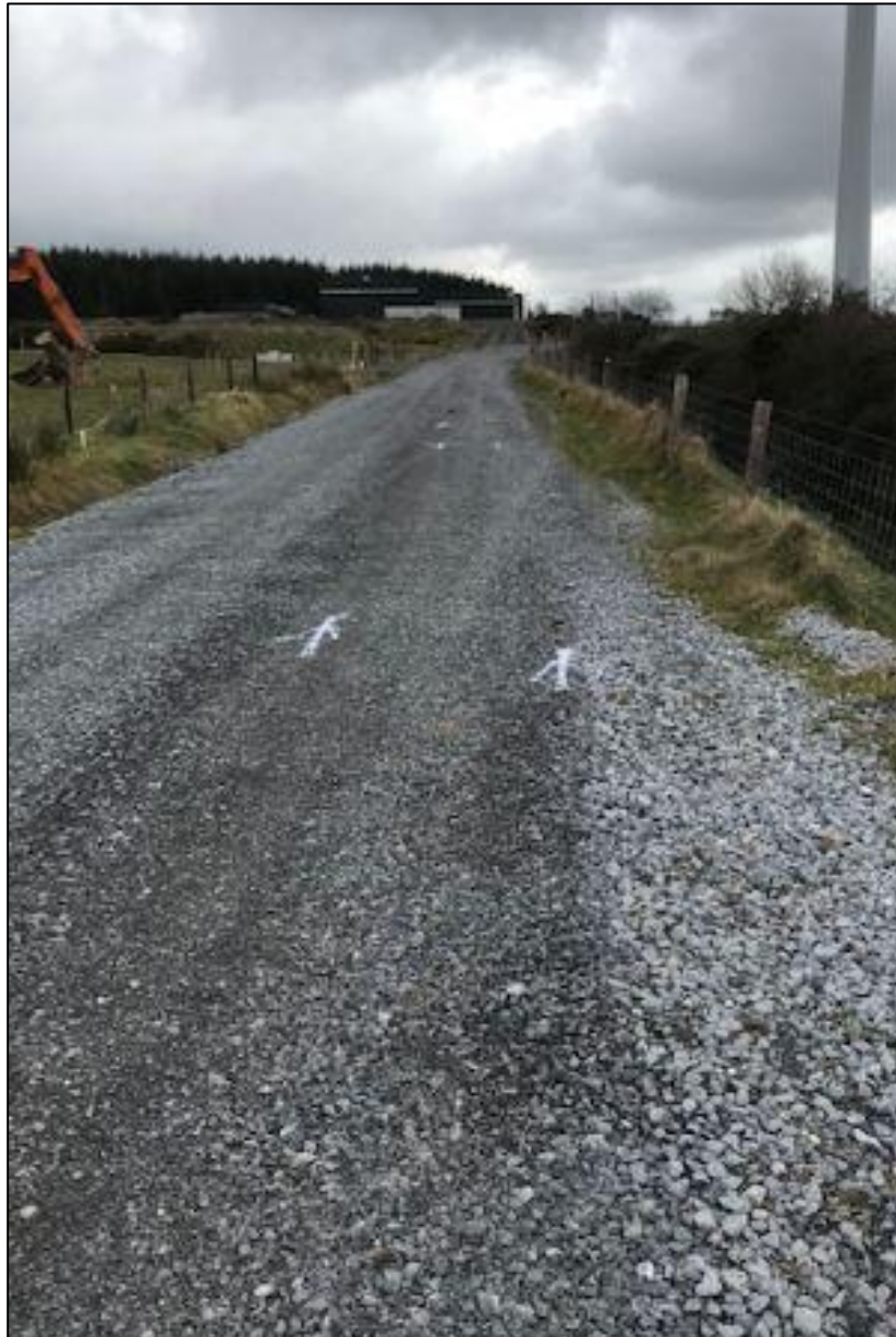
Figure 3.5: Typical Access Track
