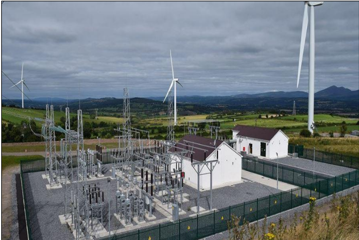
Figure 3.4: Example of a typical 110kV AIS Substation
